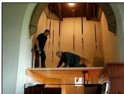
Installing the temporary ringing floor
